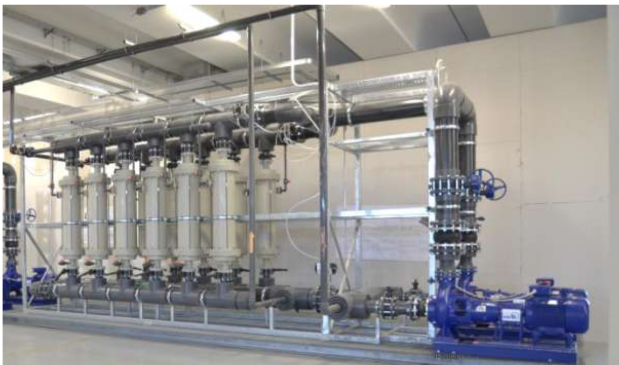
Cross-flow Wash Section
